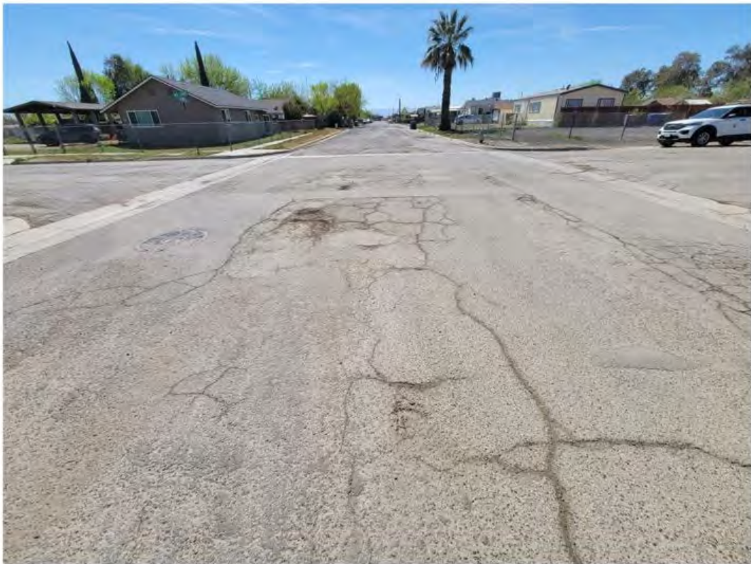
Figure 5. Daniels Ave, looking west toward Williams Ave
