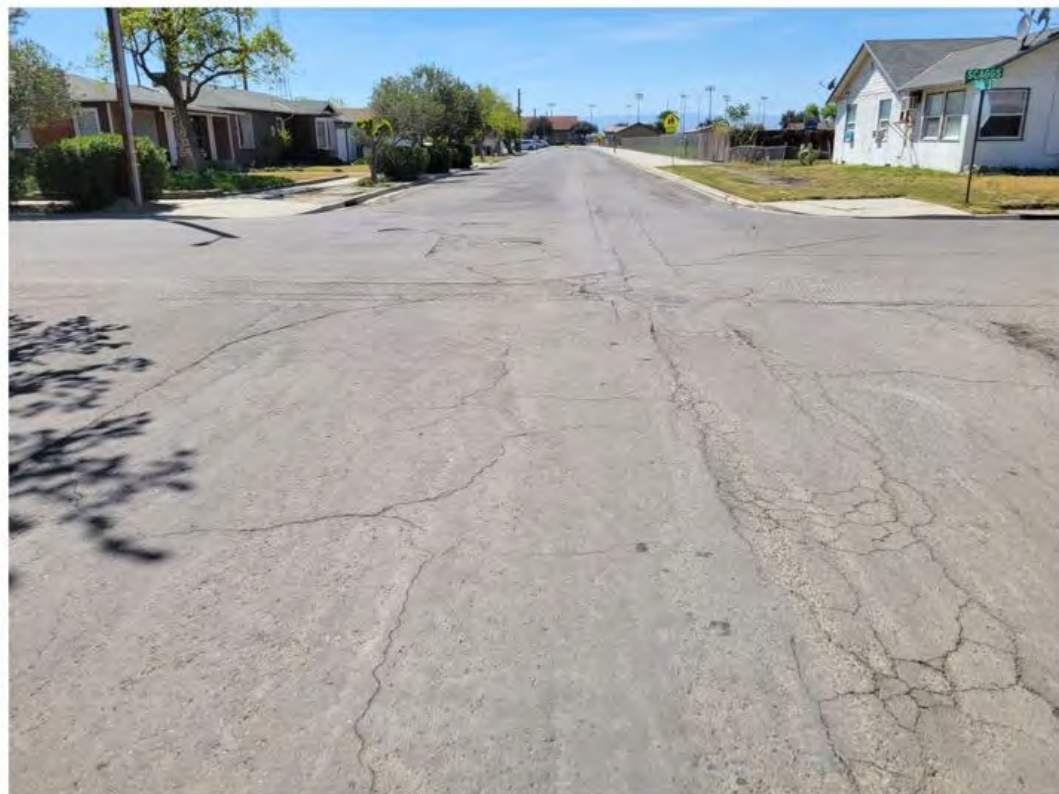
Figure 6. Daniels Ave, looking south toward Scaggs Ave
