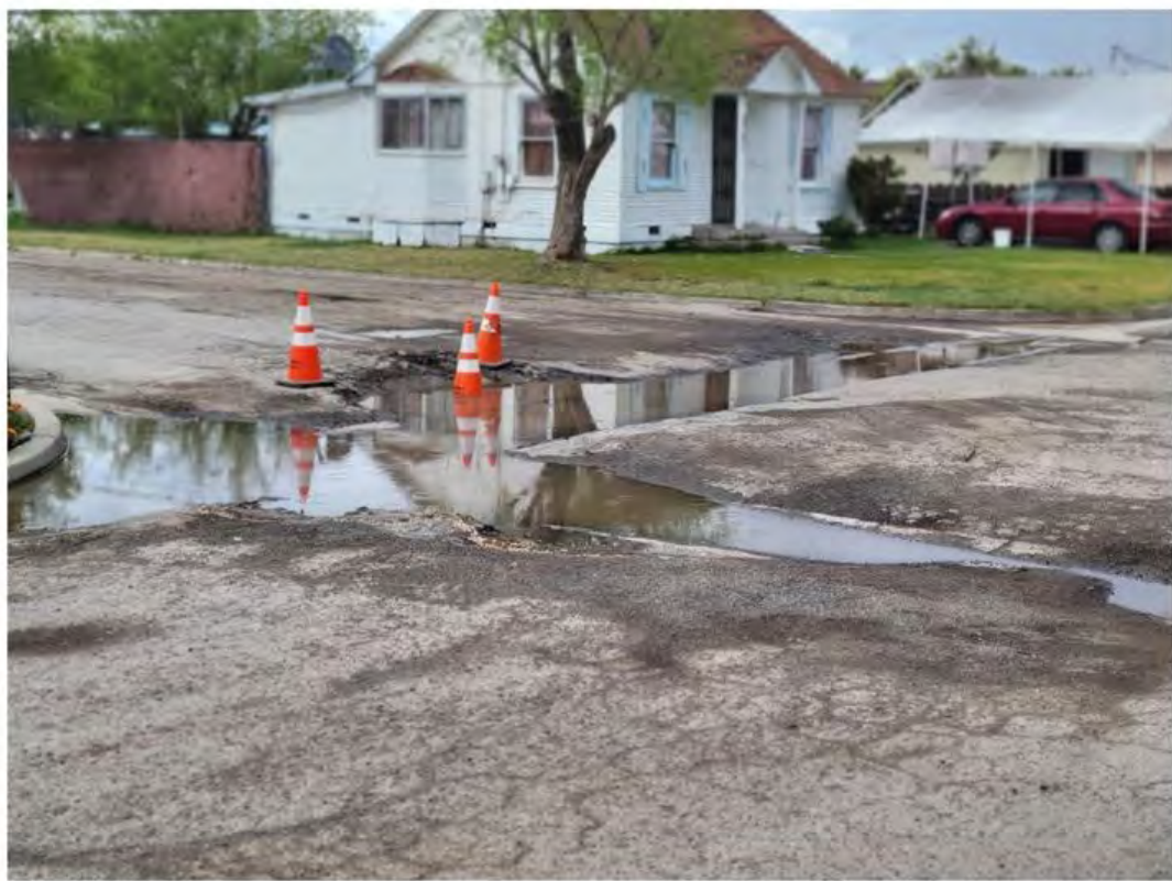
Figure 8. Anthony Ave and Williams Ave, looking northwest
