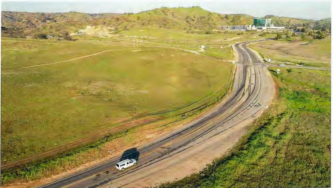
Millerton Road, just west of the new Table Mountain Hotel and Casino project, shows where the widened section of the road narrows to two lanes just as it hits a curve before continuing on into Friant. CRAIG KOHLRUSS CKOHLRUSS@FRESNOBEE.COM
