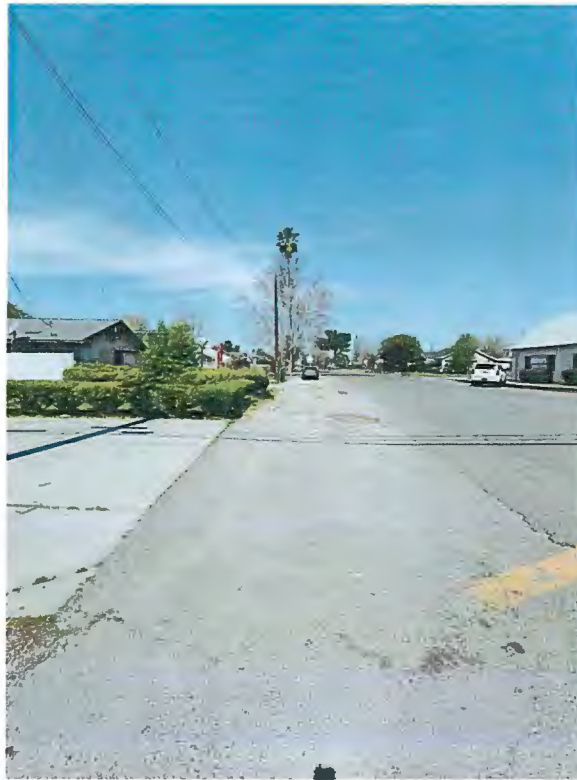
Figure 9: SW side of Quince facing NW from the NW elementary school entrance.
