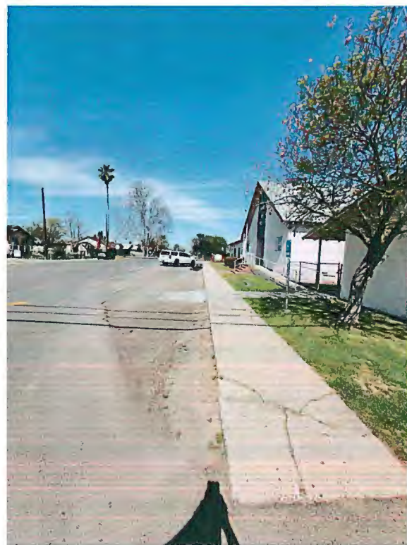
Figure 10: NE side of Quince facing NW from the NW elementary school entrance.
