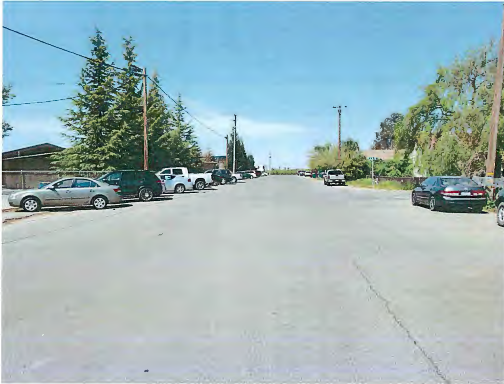
Figure 13: Raider Ave facing NW near the high school.
