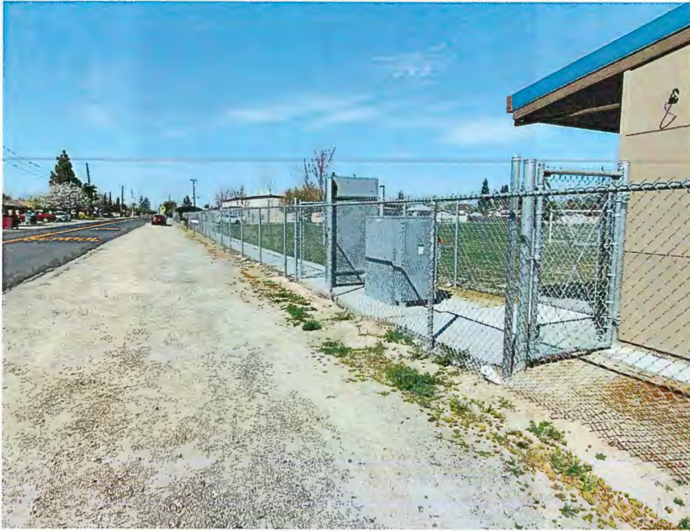
Figure 7: North side of Clemenceau Ave facing west near the elementary school.
