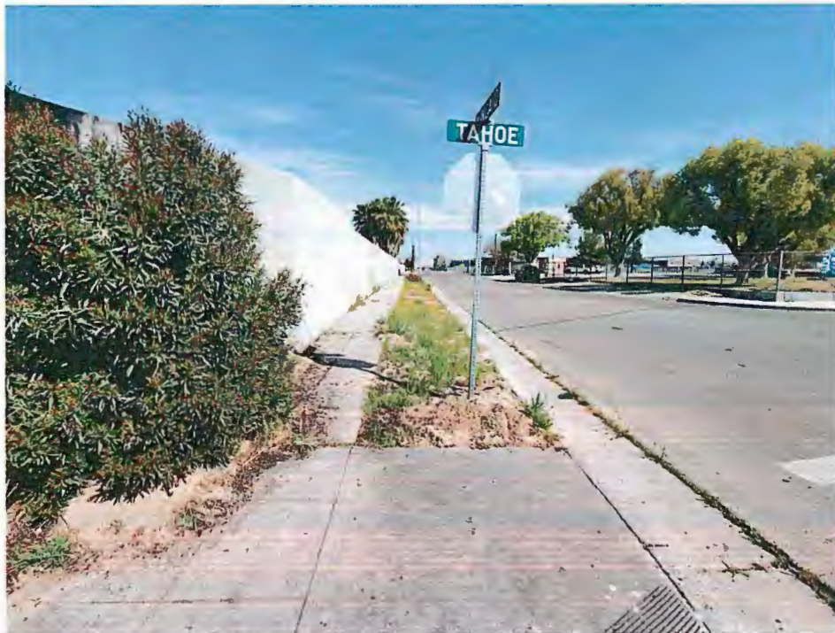
Figure 2: West side of Kincaid Ave facing north from SW corner of Tahoe Ave & Kincaid Ave near high school.
