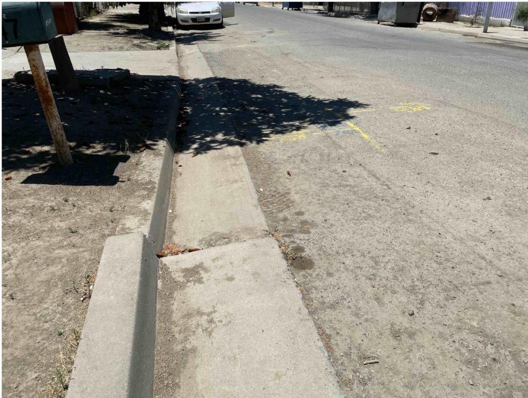
Photograph near core location C-3 – Note the differential movement in the curb and gutter
