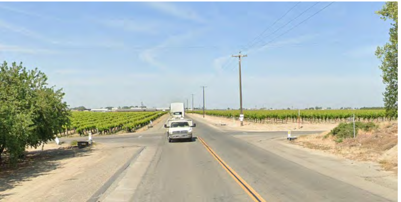
Figure 8: West Ave facing west at Manning Ave.
