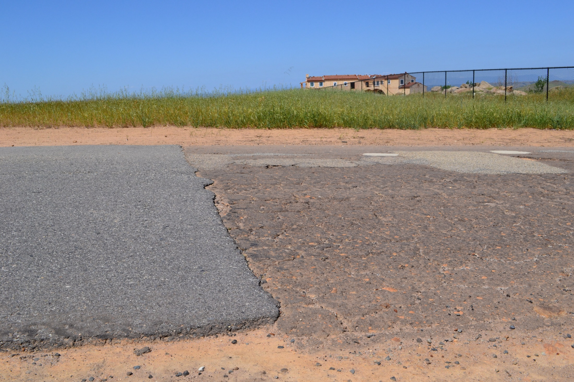
Pavement transition at the western end of the three Variances
