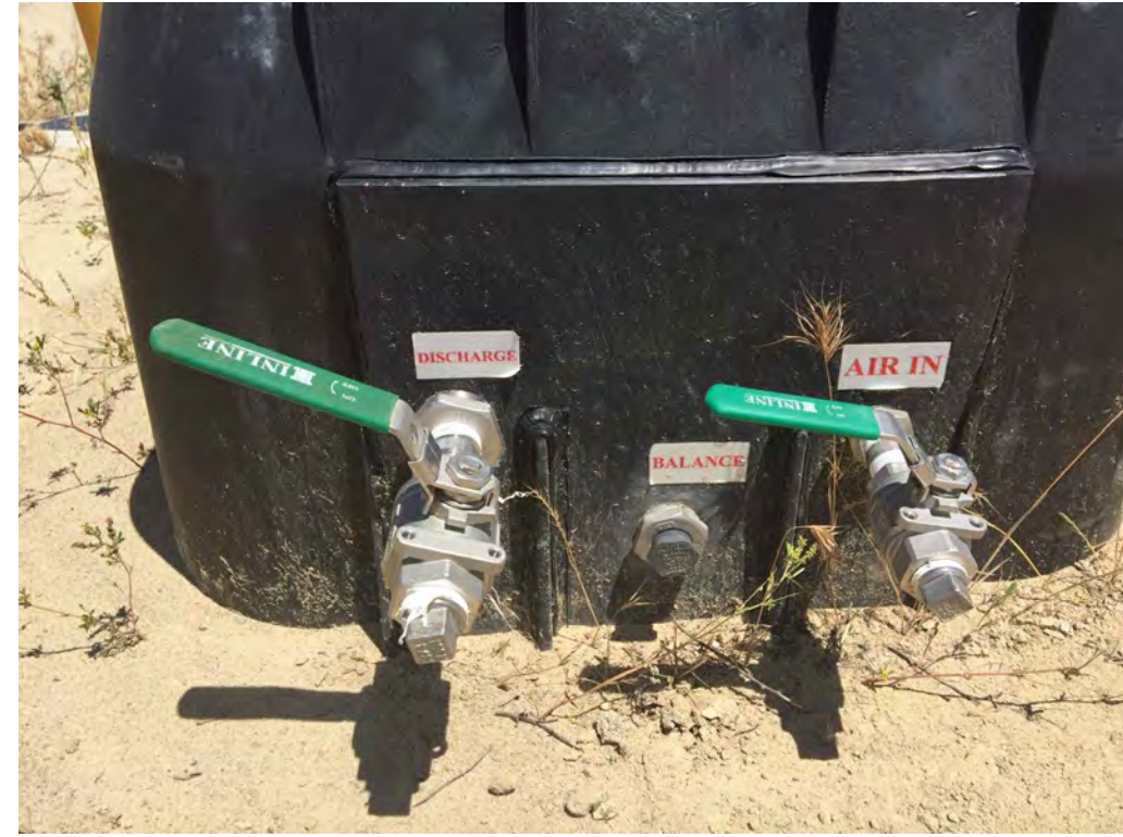
VAULT CONNECTION (WEST)
