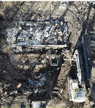
CREEK FIRE / BEFORE CLEANUP
