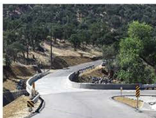
SAND CREEK BRIDGE AFTER
