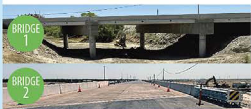
JAMES BYPASS BRIDGE REPLACEMENTS (AFTER)
