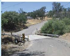
SAND CREEK BRIDGE BEFORE
