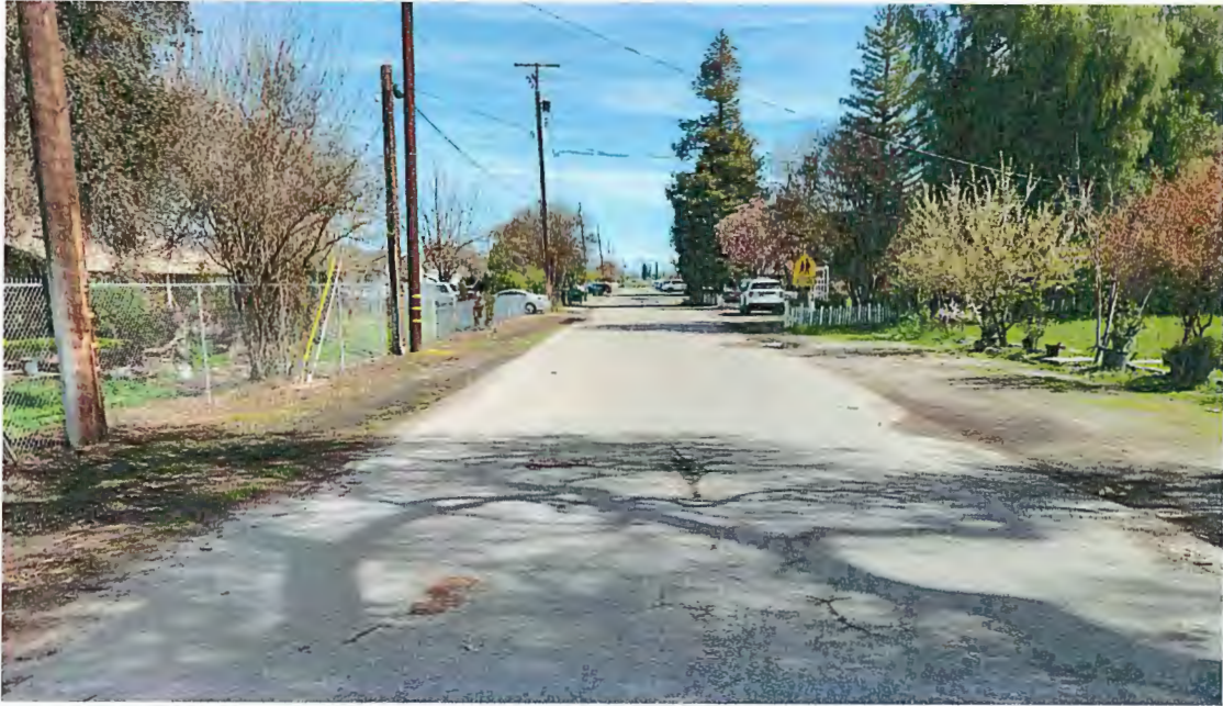
Figure 3: Willamette facing east from Elm Ave.
