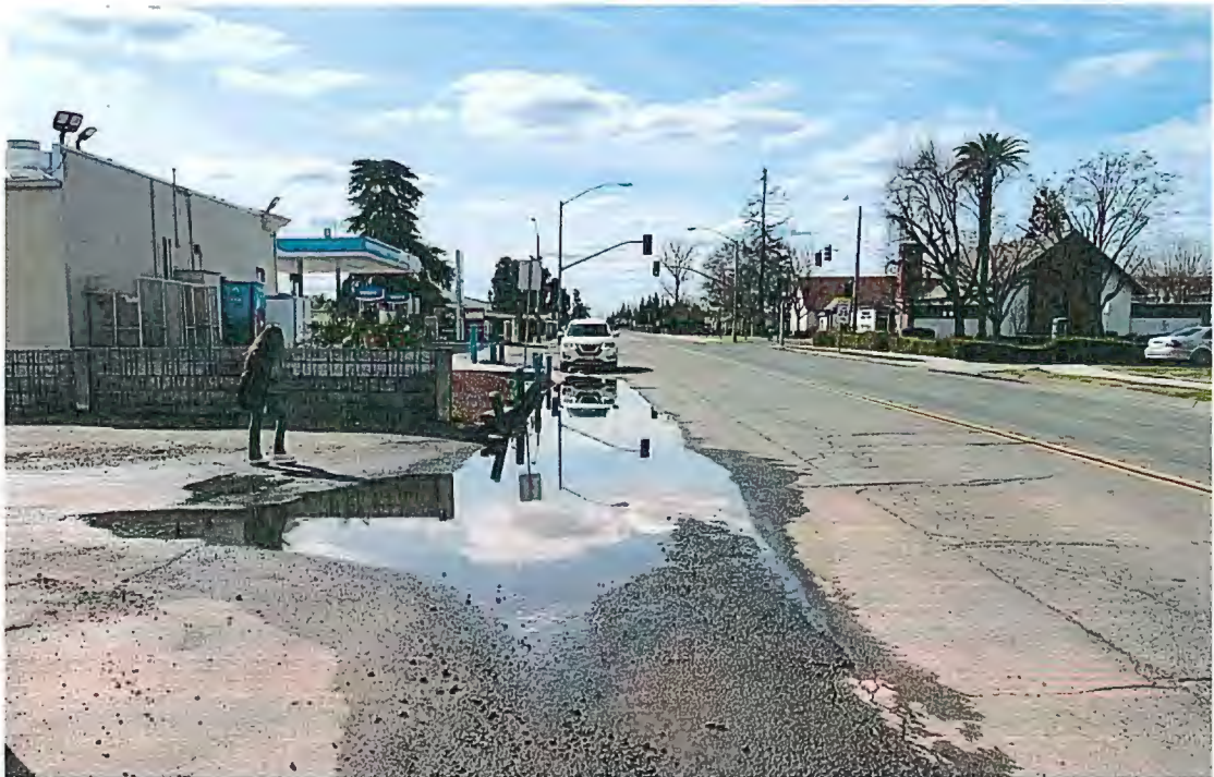
Figure 2: Student avoiding puddle on south side of Lincoln Ave near middle school.
