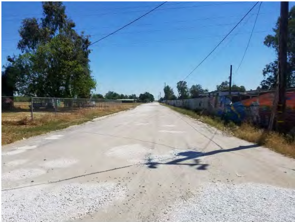
View of Northerly Road looking East in Hayes Road Community
