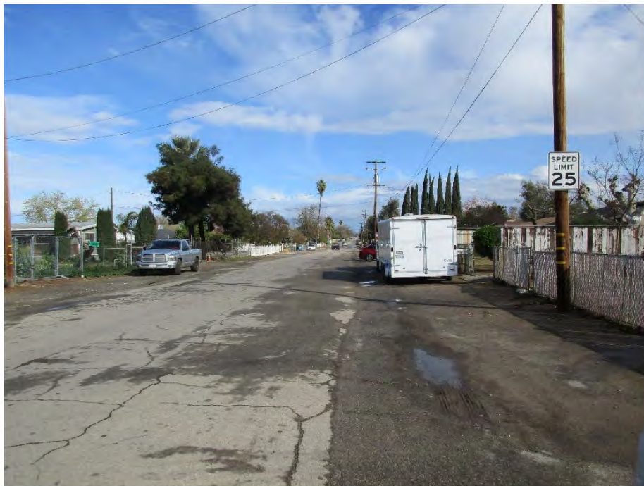
View of Prospect Avenue looking North (March 11, 2020) in the West Park Community
