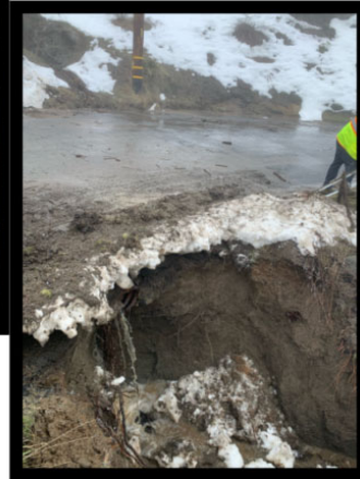
Left, Annadale Road West of Newmark suffers erosion in February 2023; middle, flooded Laton-Kingston Park in April 2023; right, erosion under Alder Springs Road in early 2023. (Fresno County Department of Public Works and Planning)
