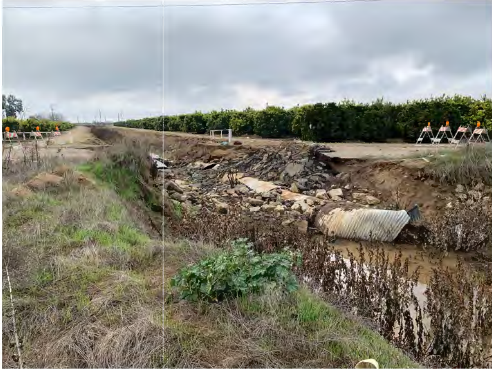
Washout due to flooding on Anchor Ave near Orange Cove in eastern Fresno County.
