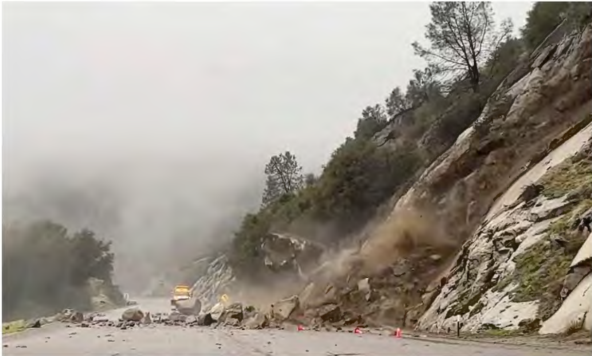
Rockslide due to storms on Highway 168 in eastern Fresno County.
