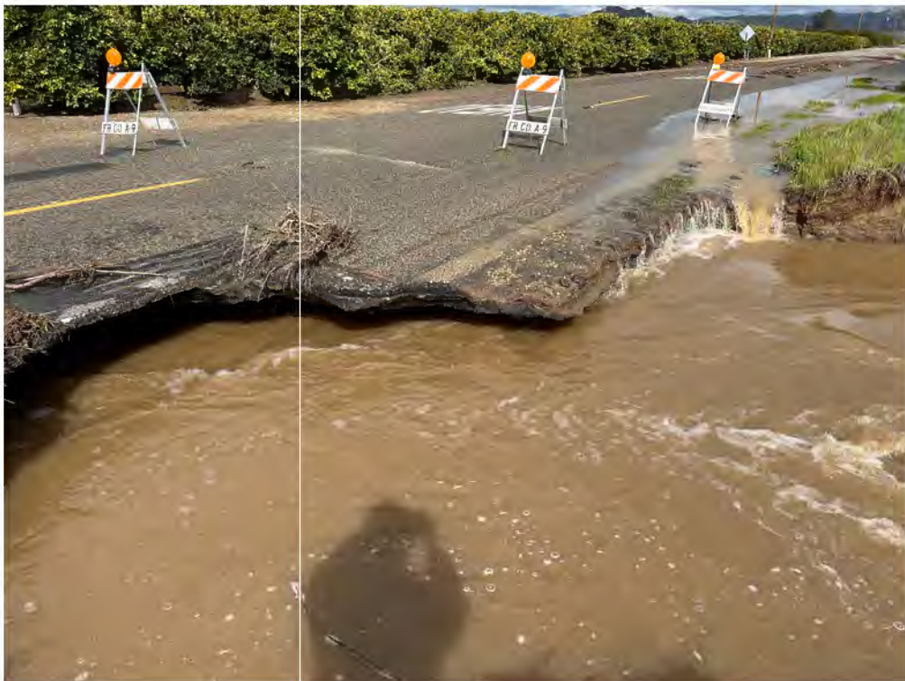
Washout due to flooding on Anchor Ave near Orange Cove in eastern Fresno County.
