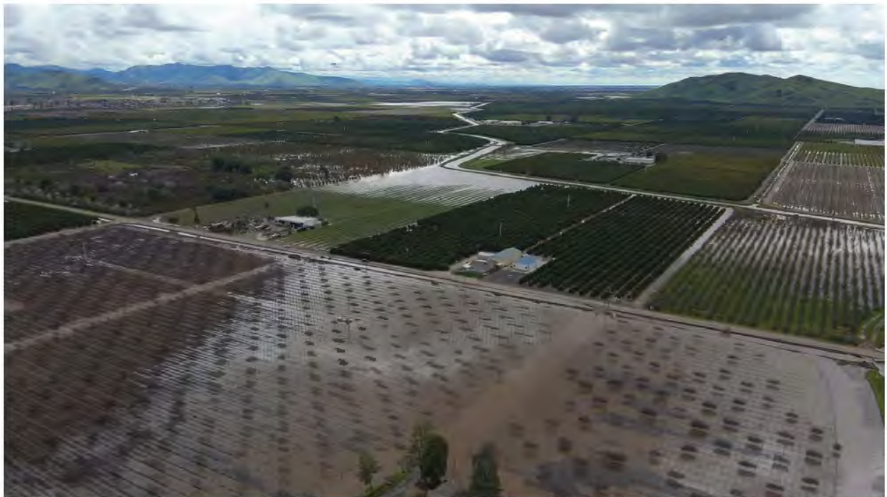
Levee breach due to storms near Sanger in eastern Fresno County.
