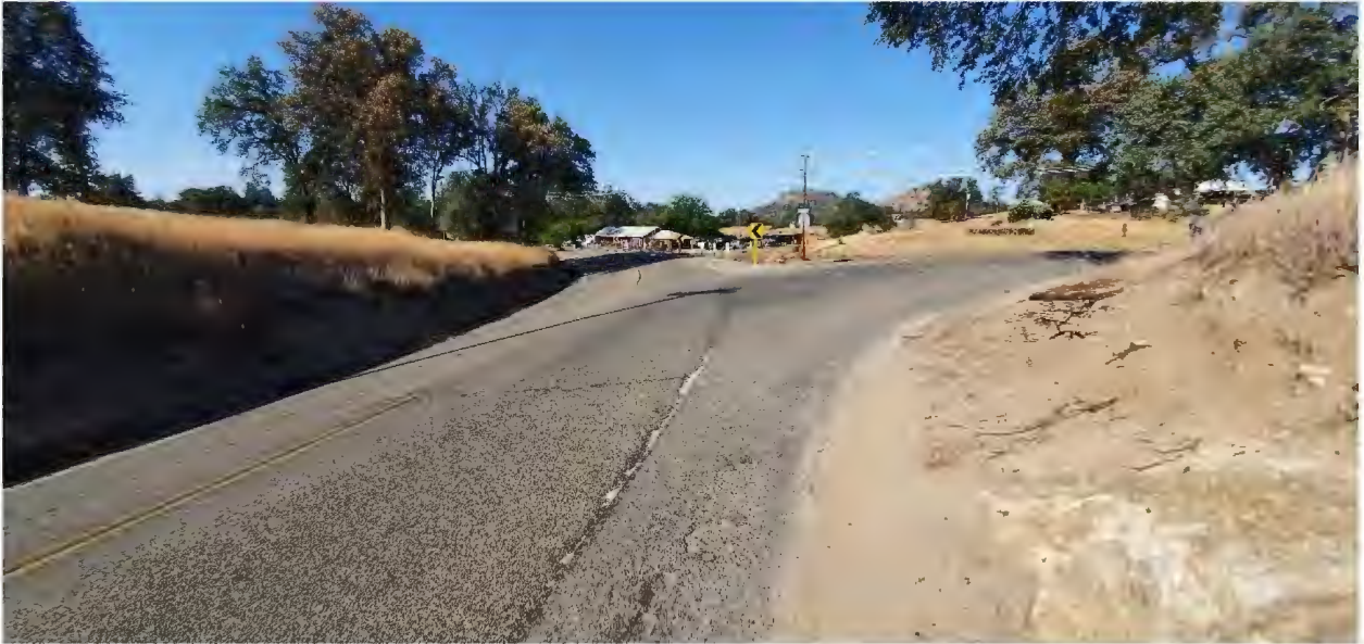
Figure 3: Looking SW at from NE side of fork..
