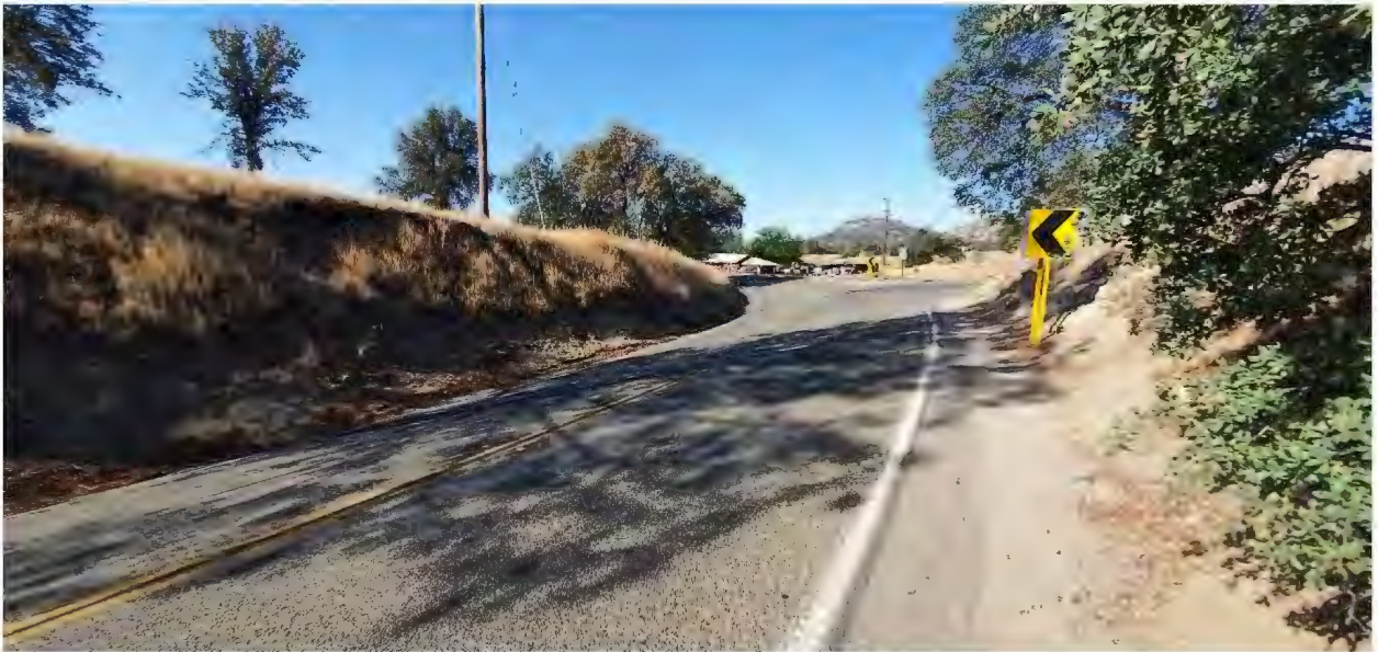
Figure 10: Looking at NE approach to Y NE from curve.
