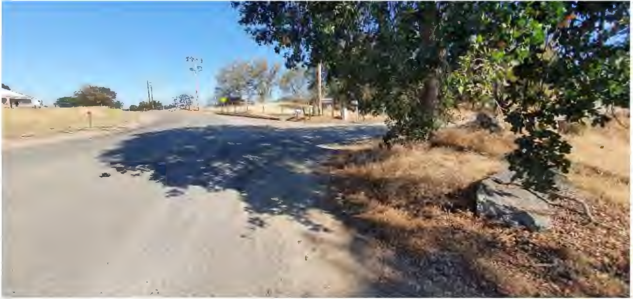
Figure 7: Looking west from NW side of fork.
