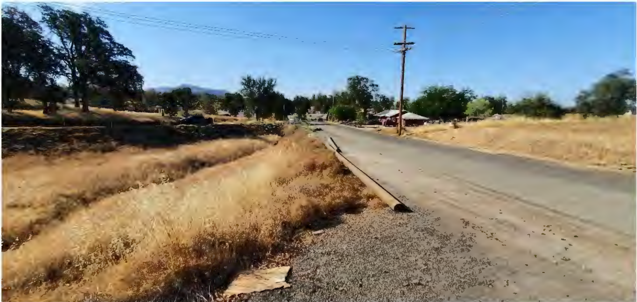
Figure 4: Looking south from northwest fork..
