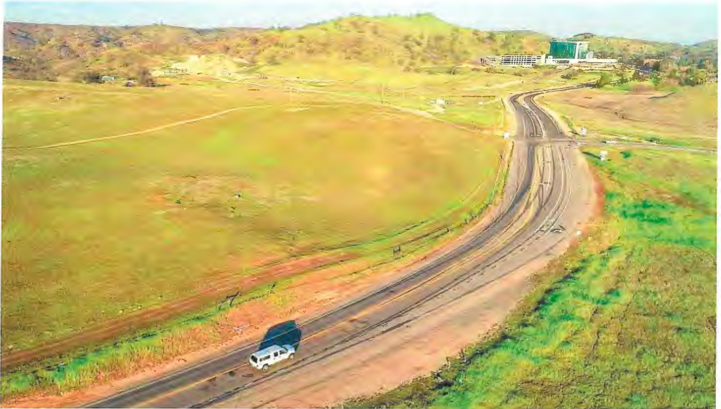
Millerton Road, just west of the new Table Mountain Hotel and Casino project, shows where the widened section of the road narrows to two lanes just as it hits a curve before continuing on into Friant. CRAIG KOHLRUSS CKOHLRUSS@FRESNOBEE.COM
